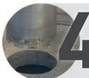
**4** | More efficient: the drilling is focused on the precise area that needs drilling. It cuts in circles, leaving a sample filling in the middle.
