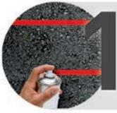
Two parallel guiding lines must be drawn on the surface to cut.
