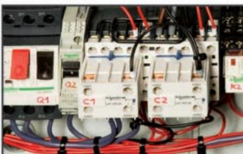
Overload magneto-thermal protection switch.
