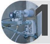
**1** | Suitable for any material: the wet core drill perforation suits all kind of materials, including green and hard reinforced concrete.
