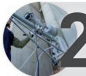
**2** | Cutting in an single pass: it can drill on concrete and steel simultaneously, without needing to change the core bit.
